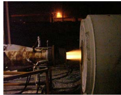
Figure 10, Combustion zone in cold oxygen mode
