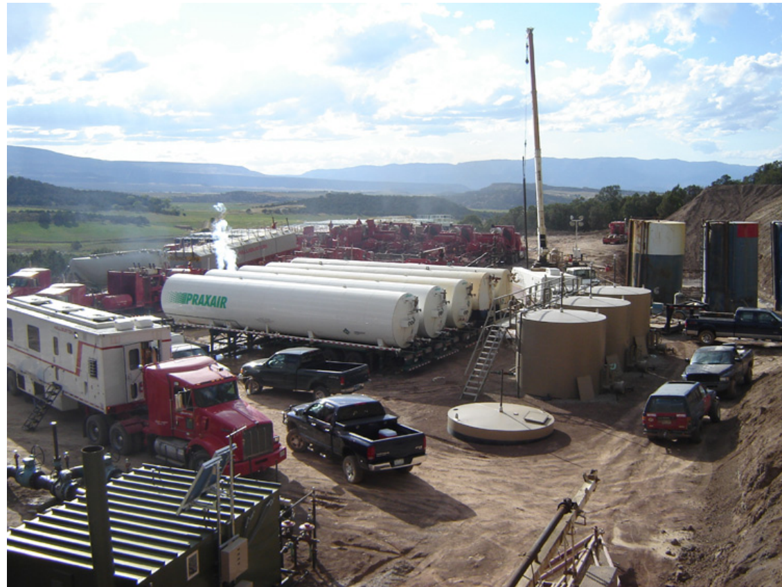
CO 2 frac job at a well in Colorado
