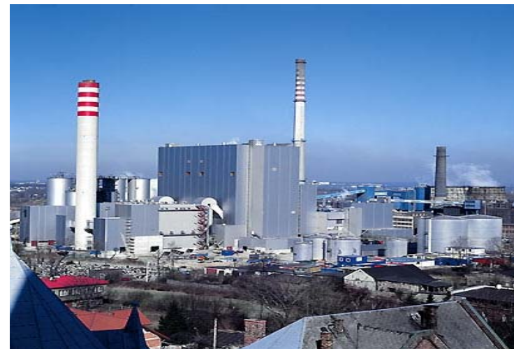
Coal fired power plant
