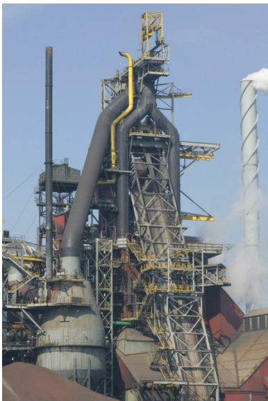
Praxair supplied Blast Furnace at USS Gary Works
