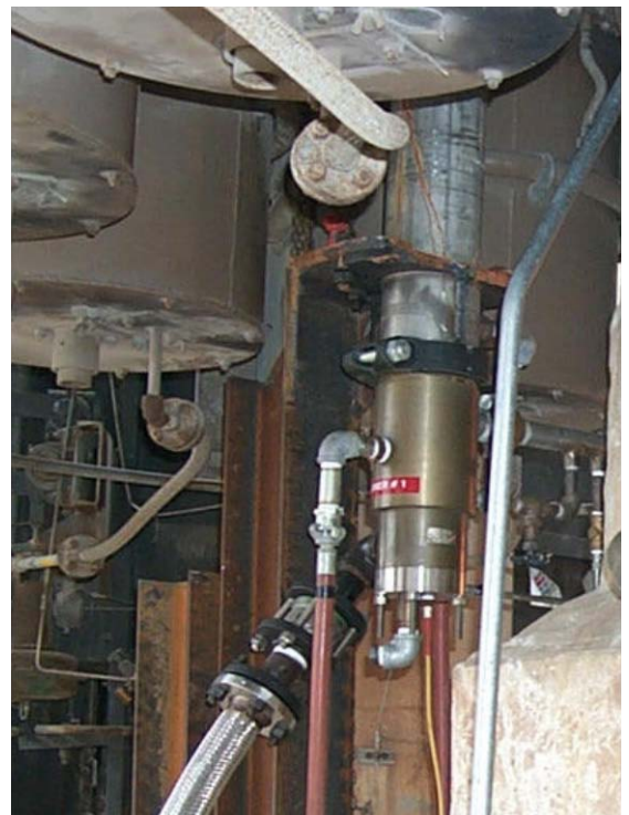
'A' Burner mounted under heater. Note size compared to air burners.
